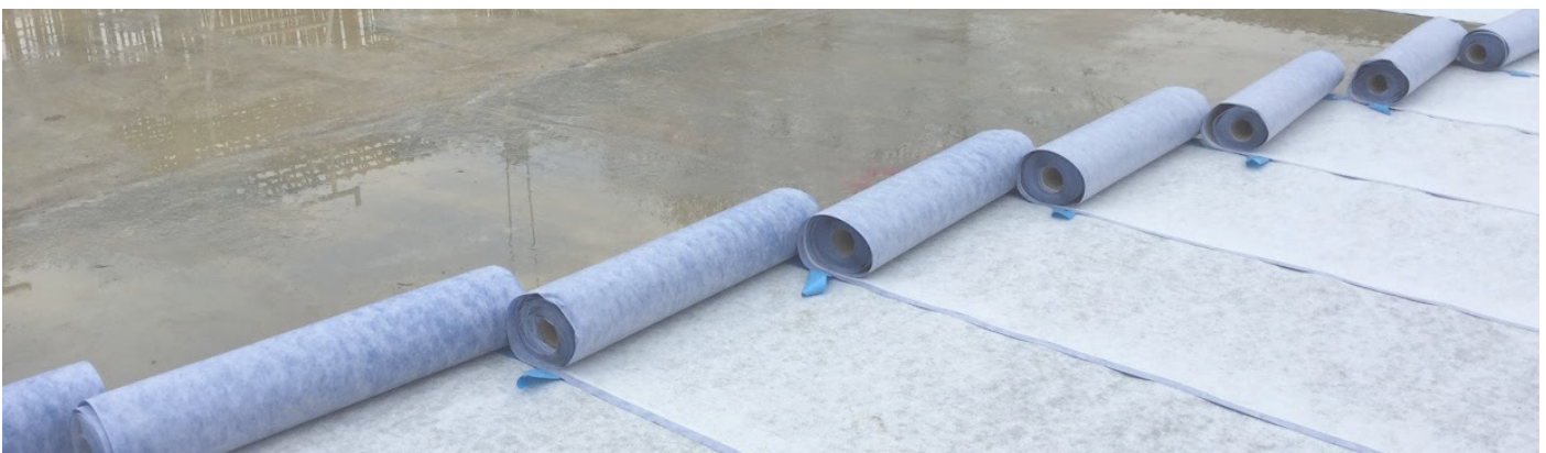
Polyfleece SX 1000 Wall under slab before casting 1x20 m.
