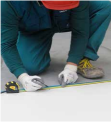
Measure, crease & fold membrane
