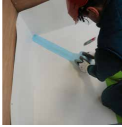
Measure, crease & fold membrane
