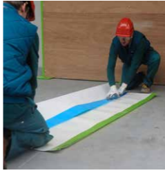
Measure, crease & fold membrane
