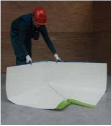
Fold internal corner & tape
